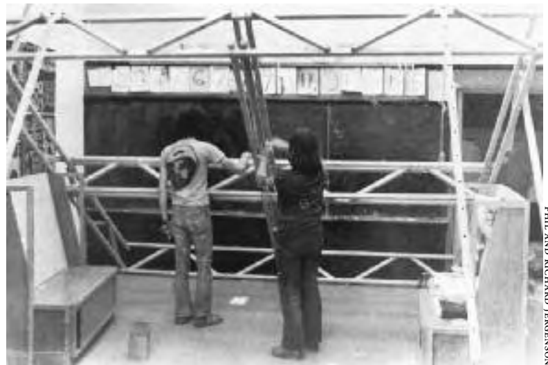
8.10: Installing a sleeping loft designed and built by Reinhold Ziegler in a preschool classroom. Truss construction keeps it strong and light.
