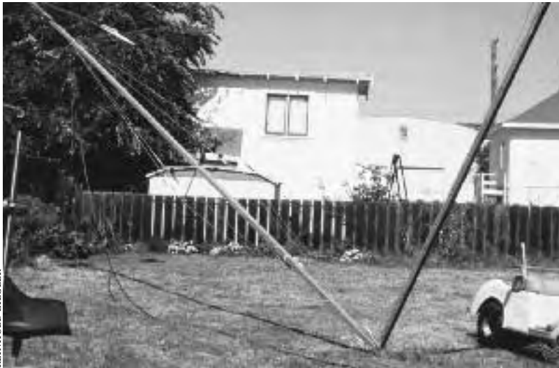
9.6b: Raising the 40-foot (12-meter) tower using the gin pole.
