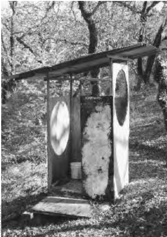
8.11: Grid beam outhouse built by Richard in 2006. The frame is damaged 1½-inch wooden sticks, with sides of reused plywood and a roof of scrap Alucobond. The panel with the round hole was recycled from Phil's Portable House.
