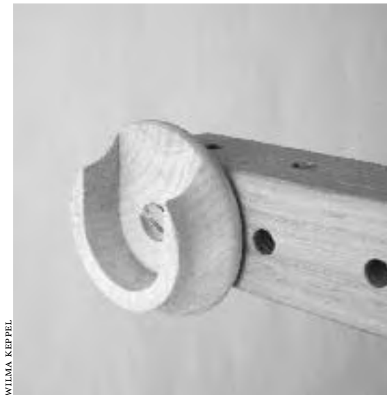
15.15: Wooden clothes pole support on Richard's free-standing closet attaches with a tapered machine screw and weld nut.
