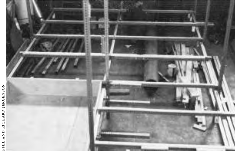
8.14: Kent built the frame of his Tent House inside the Earthlab I warehouse in Berkeley. The recessed kitchen floor at left fits under the sleeping loft.
