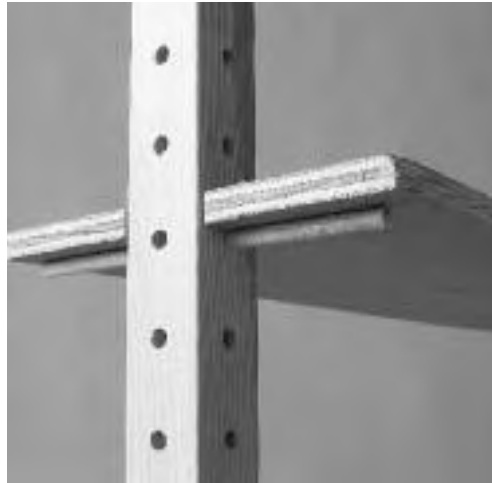
15.12: Wooden dowels support a notched shelf on the Conversation Lounge.
