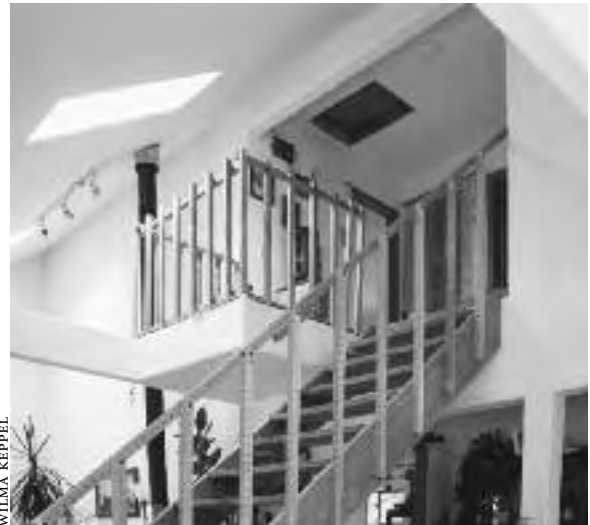
8.4: Phil put up this wooden stair railing in about an hour. It lag screws to the stairway. The balcony railing screws to the floor through the carpet.
