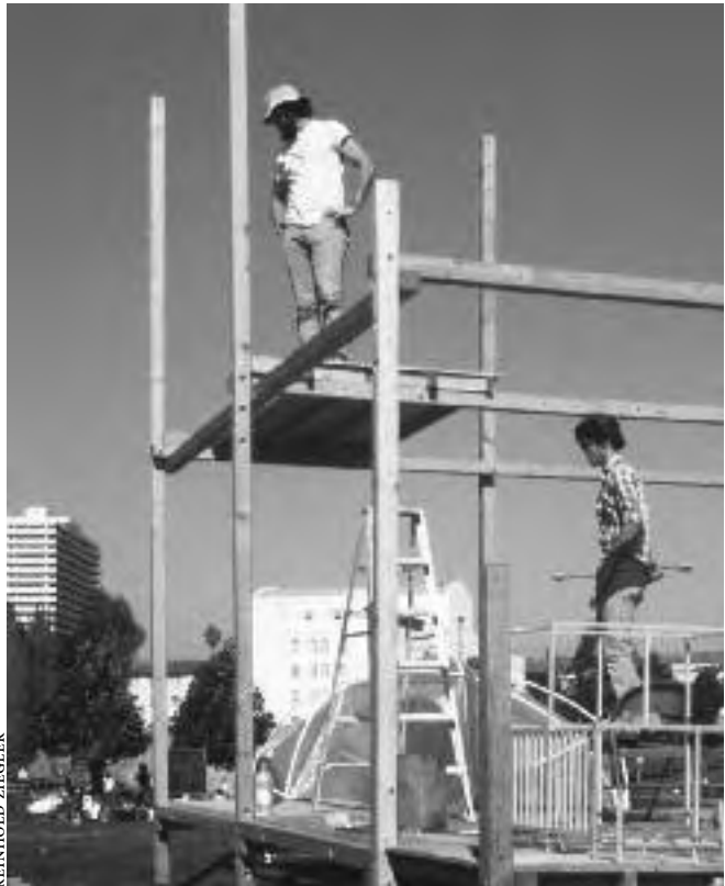
2.10: Students assemble a solar cabin, framed with wooden four-by-fours measuring 3½ inches square, for a 1980 college fair in Oakland, California. Design by Reinhold Ziegler.
