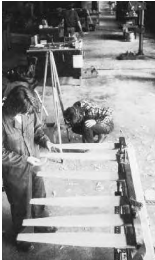
7.14: Tom Conlon’s clamp for making wind turbine blades. Frame is 2-inch steel tubes that Tom drilled every 1 inch.
