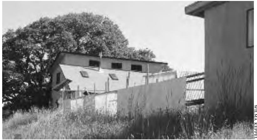
13.9: Phil's steel-framed yard fence has a mix of corrugated steel and fiberglass panels.
