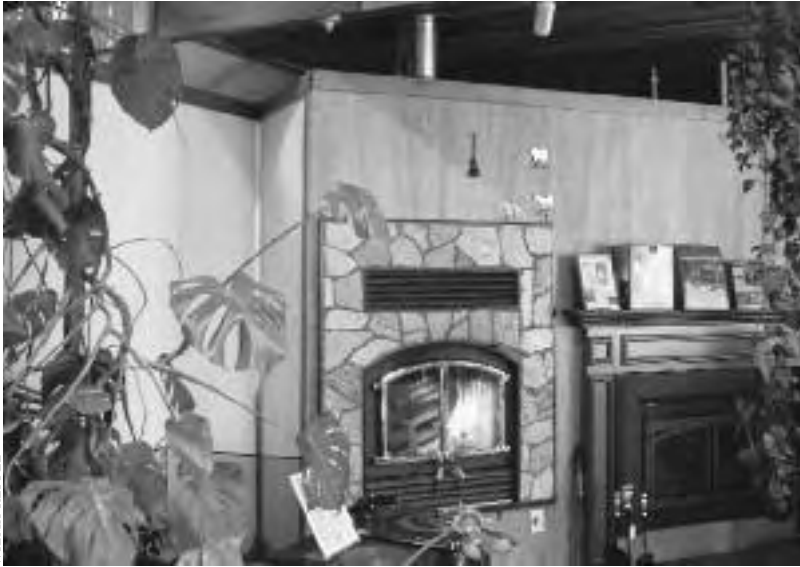
8.7: Fireplace display wall in Earthlab Energy Systems’ Willits showroom. Built of plywood on a frame of 2-inch galvanized steel, the wall lag screws to the building frame.
