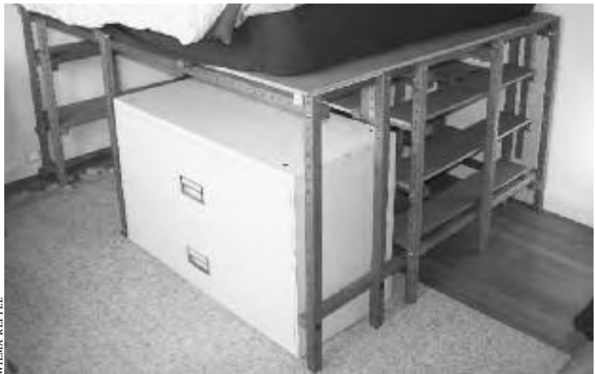
3.3e: L-shaped space under Version 4 platform lined with 50 feet of bookshelves, with room to sit up comfortably. White bathroom paneling bounces light from the ceiling and end.
