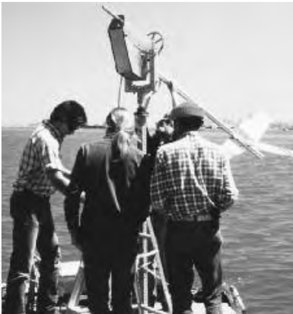
2.9: Reinhold Ziegler used grid beam in the wind and solar energy classes he taught in California colleges starting in 1979: "We never needed to weld one part in 7 years of classes." Here students install a steel-framed windmill and stand, which they designed and built, on a floating platform in San Francisco Bay.
