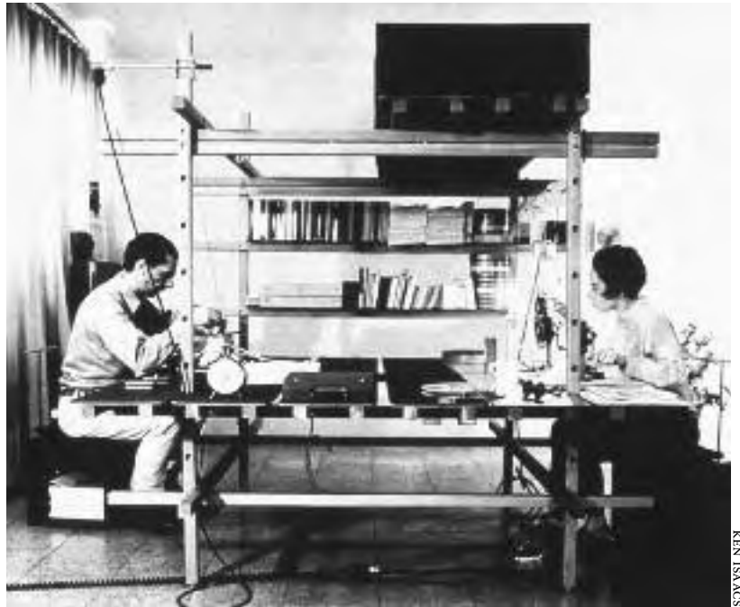
5.15: Living Structure in Ken Isaacs's Chicago apartment. Movable hardboard pallets make a table, seats and an overhead storage platform.
