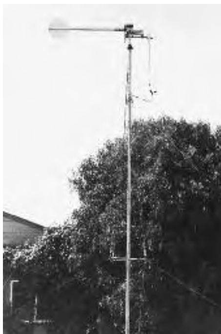
9.1: Tensioned cables brace a wind turbine tower made of 2-inch galvanized steel, built by students in Reinhold Ziegler's 1980 alternative energy classes. The grid beam turbine generates electricity.
