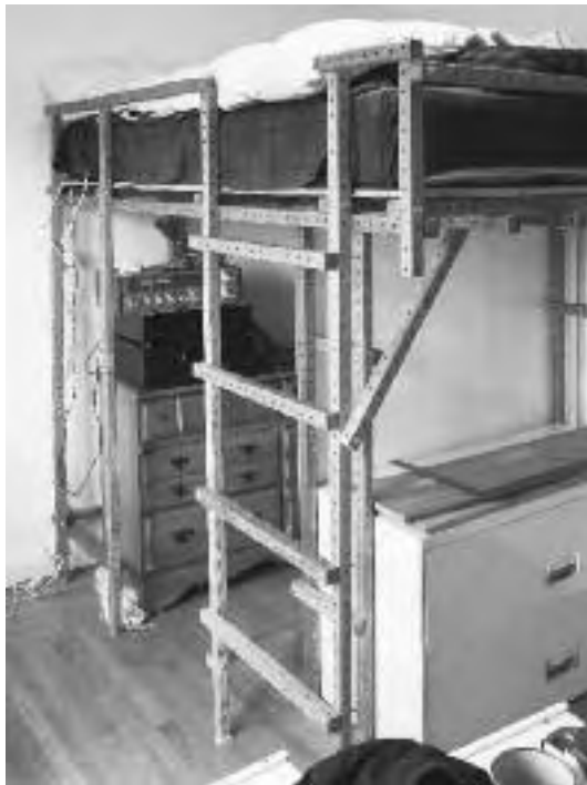
3.3a: It usually takes about three tries to get a project the way you want it. The first version of Wilma's bed loft wasted floor space. The panel behind the file cabinet made the room seem cramped.
