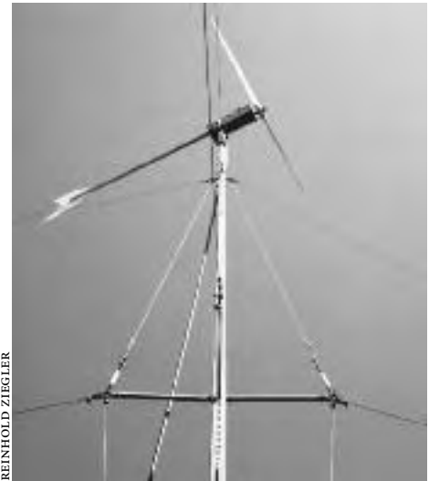
9.6c: Tower installed. Cables stiffen the mast and keep it vertical.
